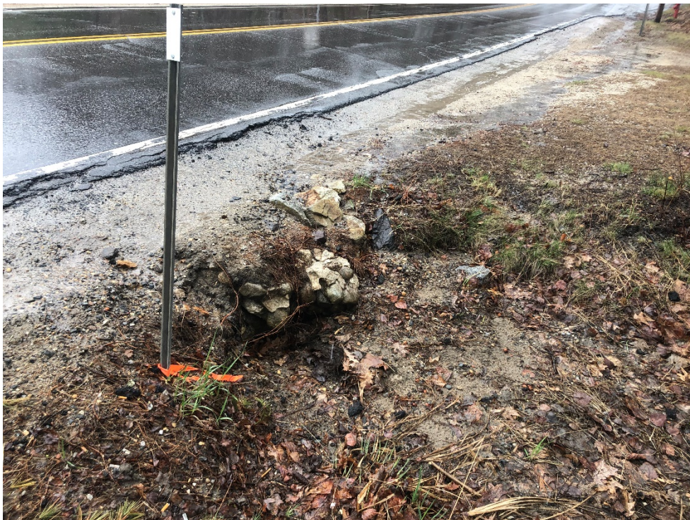
Photo 10. Shallow depression conveys stormwater from Frank C Gilman Hwy to Mill Pond.
