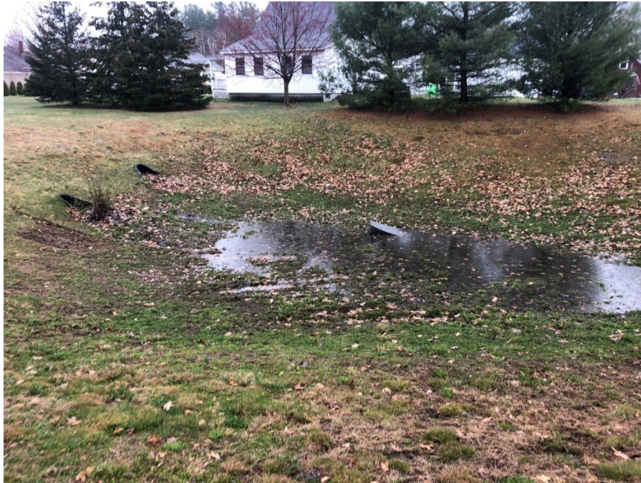
Photo 3. Retention pond at Profile Bank manages stormwater for DA3
