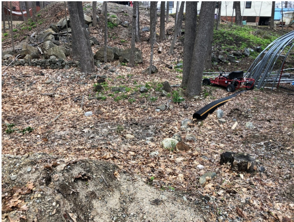
Photo 4. Outfall 4 is directed to a natural depression via a pipe.
