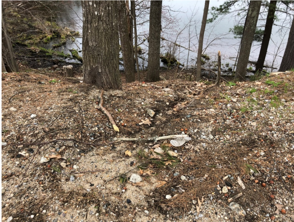
Photo 5. Channel gully forming at top of bank flowing towards Mill Pond.
